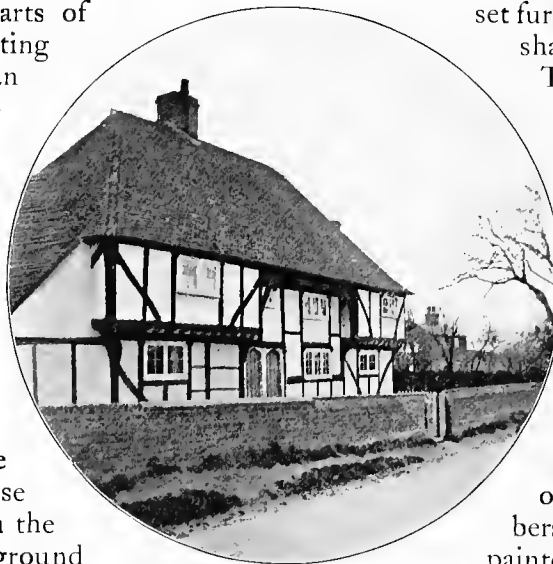
OLD COTTAGES AT BOUGHTON-UNDER- BLEAN, KENT
